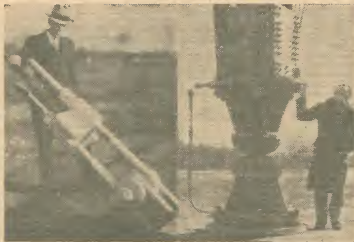
Here's one of the guy anchors (left) and the insulated base (right) of America's tallest broadcasting antenna. The steel lattice-work tower is that of WSM, at Nashville, and rises RGR feet into the air. WLW, at Cincinnati and other new 50,000 watt stations have likewise adopted this type of "vertical radiator."
